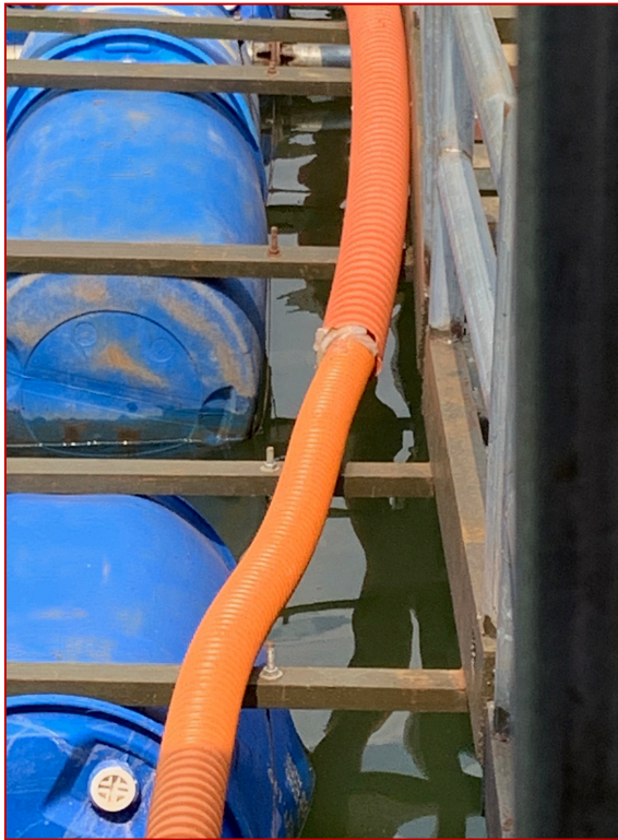
Figure 3-11: Electrical cable cover was not considered safe
