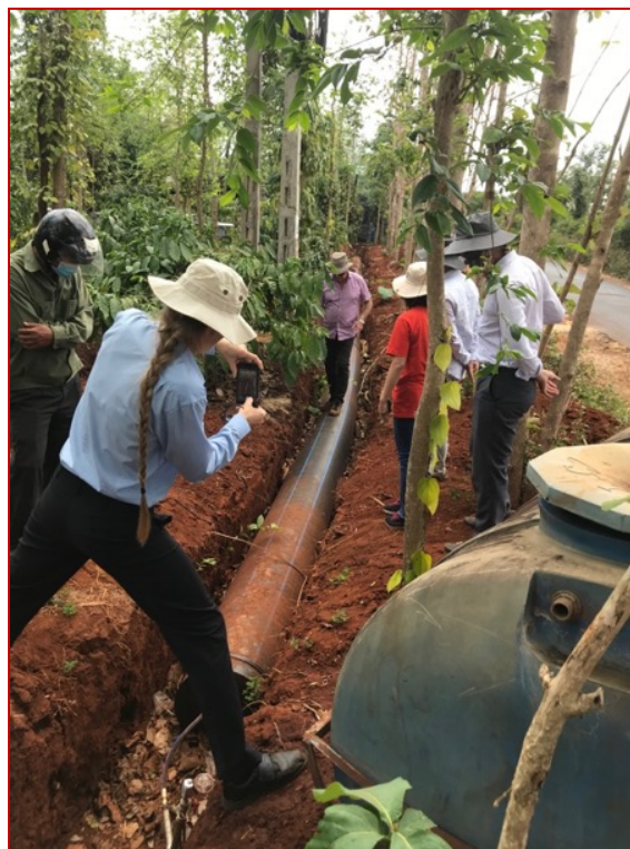
Figure 3-3: Inspecting the alignment of the pipe – showing insufficient clearance on both sides of pipe
