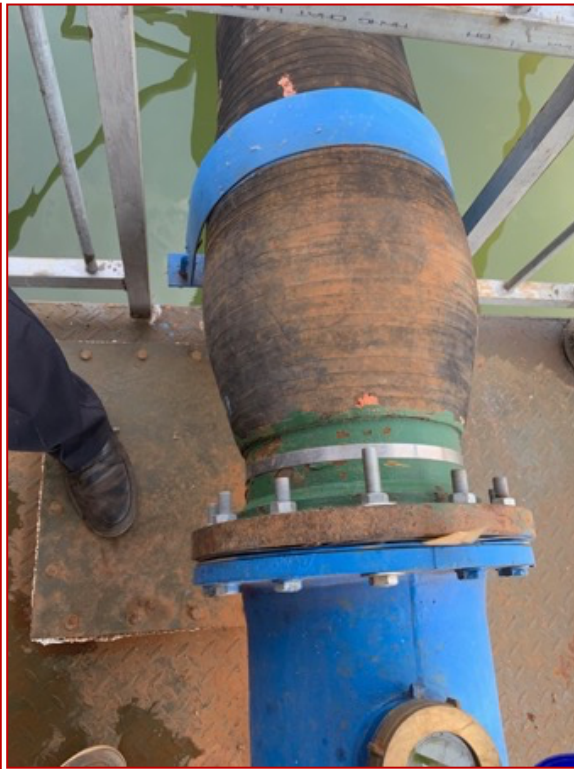
Figure 3-10: Showing the fittings already expanding and in danger of collapse
