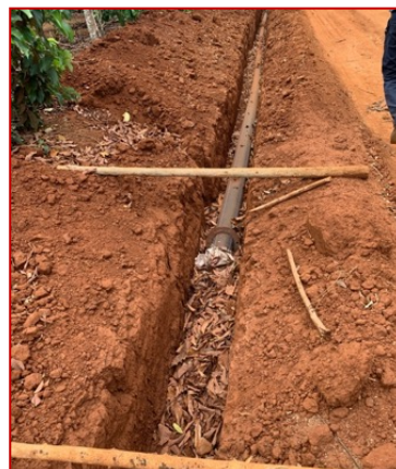
Figure 3-5: Offtake structure – the offtake pipe should have connected upstream on the larger pipe to enable better pipe flow efficiencies
