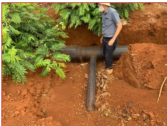
Figure 3-6: Showing the debris around the pipe
